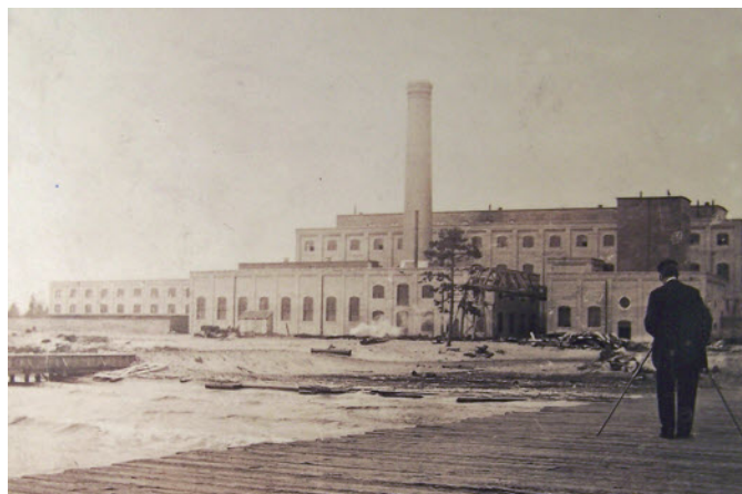
In 1903, the Tawas Sugar Company constructed this processing plant at East Tawas, southwest of today's Tawas Beach R. Road "Y" intersection with Huron Shore Road. The plant closed in 1905 because of a lack of beets to process.
