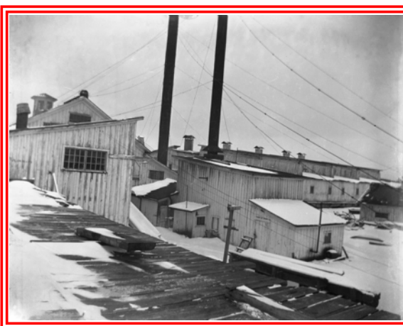
This mill complex owned by Temple Emery housed the National Milling and Evaporation Company at East Tawas. The old lumber mill was modified and remodeled for its new purpose of processing potatoes.
